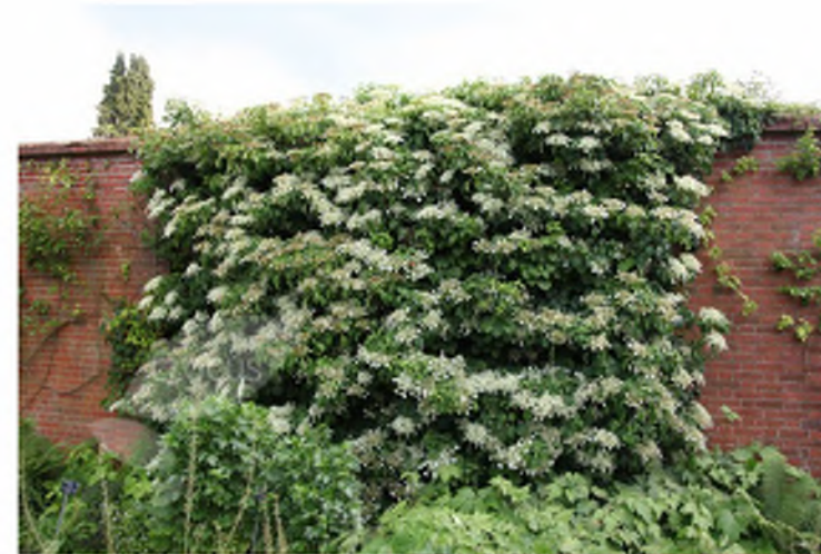
NORTH GREENROOF WALL AND HVAC SCREENING
